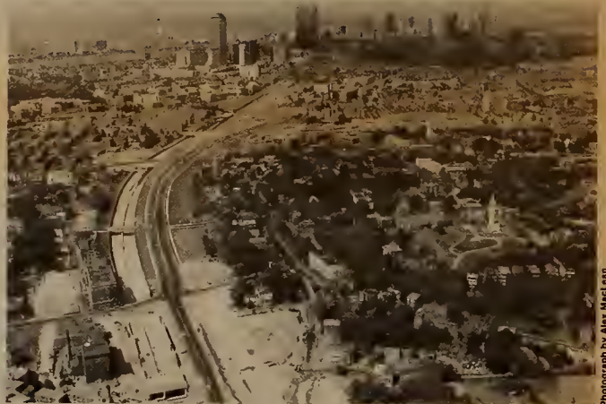
Section II of the SWCP, with Downtown Boston and Section I in the background.
